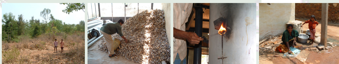
In the village of Hosahalli, Tumkur district, Karnataka state in southern India, a biomass driven energy system has been under operation since 1988. The system is based on a standard diesel engine generator system. The fuel is, however, provided through a biomass gasifier. A plot of 4 ha, about 1 km from the village, planted with fast growing tree species provides the biomass needed. This system has the potential of reducing the consumption of fossil fuels by a long-term average of 75 percent. The system generates electricity for lighting, irrigation, drinking water and services such as the milling of grains.
