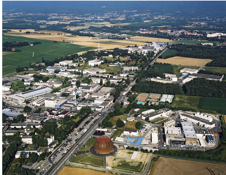
Fig. 14. Here I could imagine an picture of the present ISOLDE with arrows pointing to the new buildings. For HIE it would be the hall extension. This needs, however, that we send up a brave man or woman in a crane for a nice photo. And maybe nice wether.
